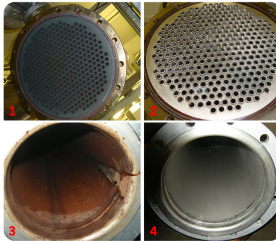
Fig. 2. Tube plate of a steam raising unit before (1) and after (2) derouging. Pipe system before (3) and after (4) rust removal with new pH neutral formulations with NTZ clean neutral .
