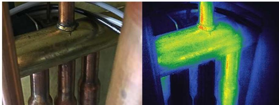
**Figure 6. Thermal photo taken during the diagnosis of faulty valves**
